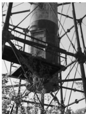
Access door to steel tower. Missing catwalk to fog signal building.
